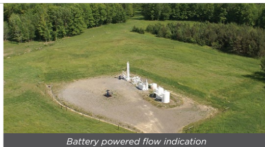
Battery powered flow indication
