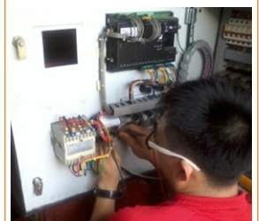
Mounting an F116 into a panel
