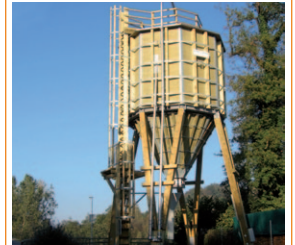
8-sided wooden silo
